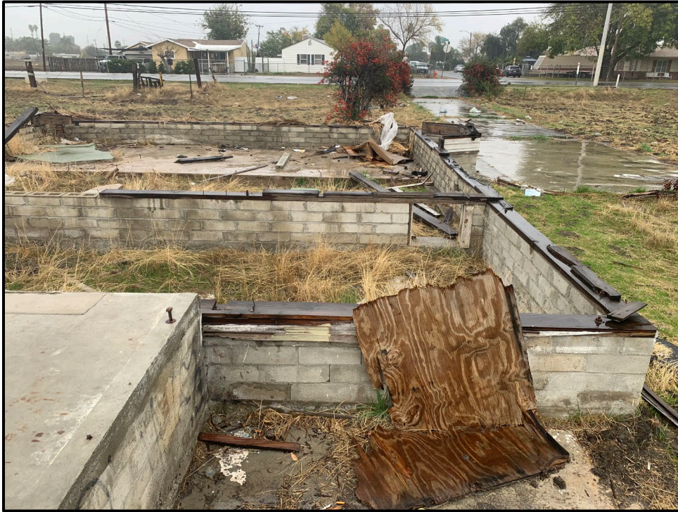
Plate 3.2–16: Overview of the foundation for the single-family residence, facing east.
