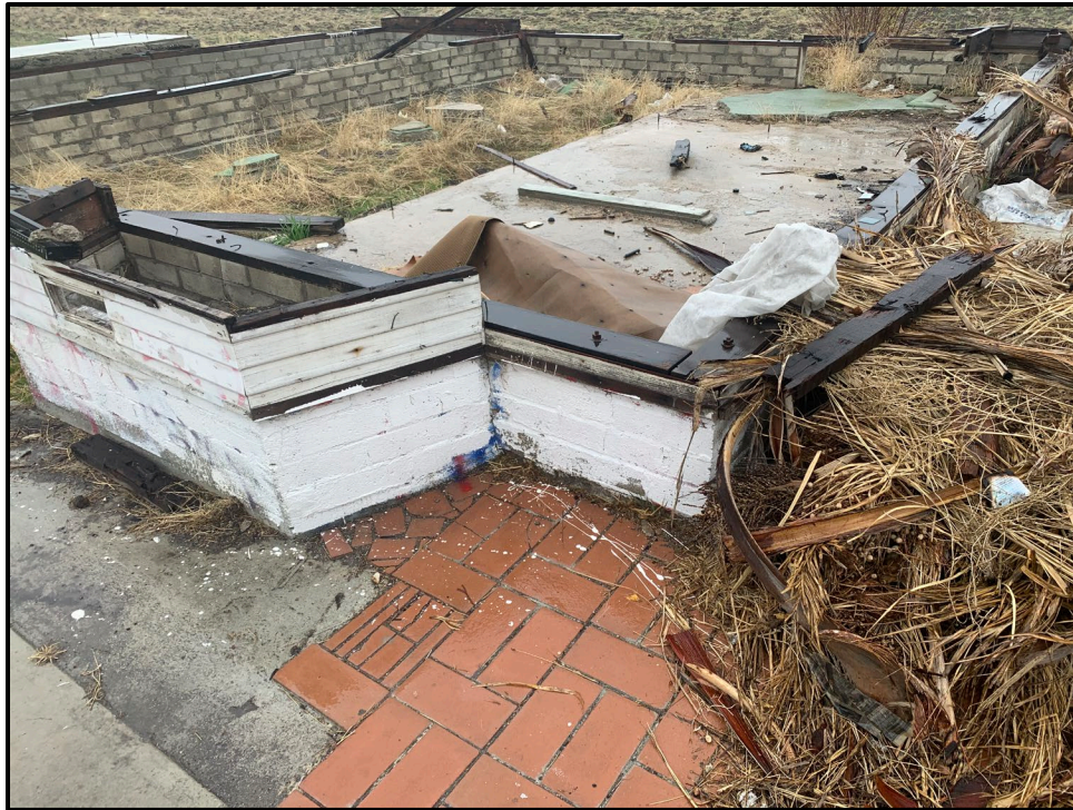
Plate 3.2-18: Overview of the foundation for the single-family residence, showing the bay window, facing northwest.
